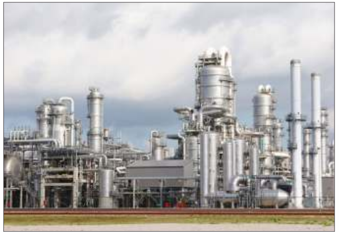
De-watering for chemical industries
